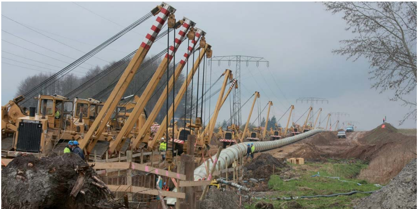
Moving into a Microtunnel DN 2200 with sliding skid
