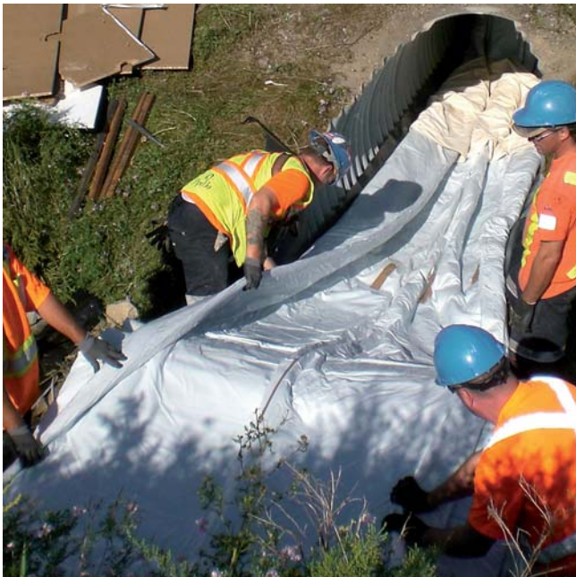
Installing the DN 1,200
