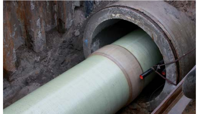
Moving into a Microtunnel DN 2200 with sliding skid
