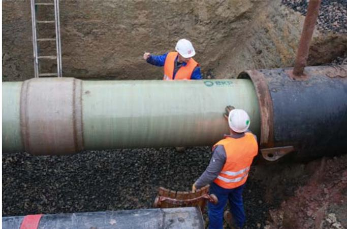
**Casing tube DN 1,200 (black) – BWB-coated steel pipe (green) with GRP-spacer (brownish)**
