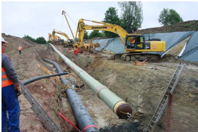
**Holding the 90 meter long pipe section in right position**
