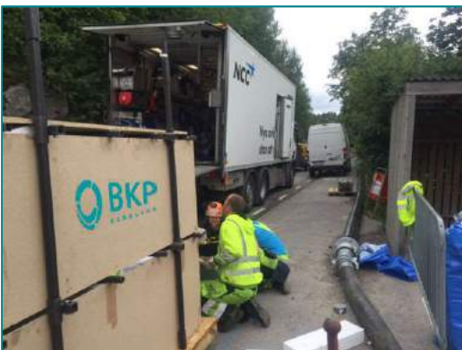
Installation using DN5 500 for 200 meter rehabilitation - Botkyrka, Stockholm.
